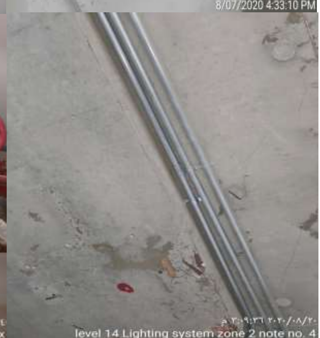
level 14 EIB/KNX 2nd fix
